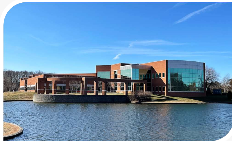
RCKT Cranbury (NJ) 103,720 sq. ft. production facility
